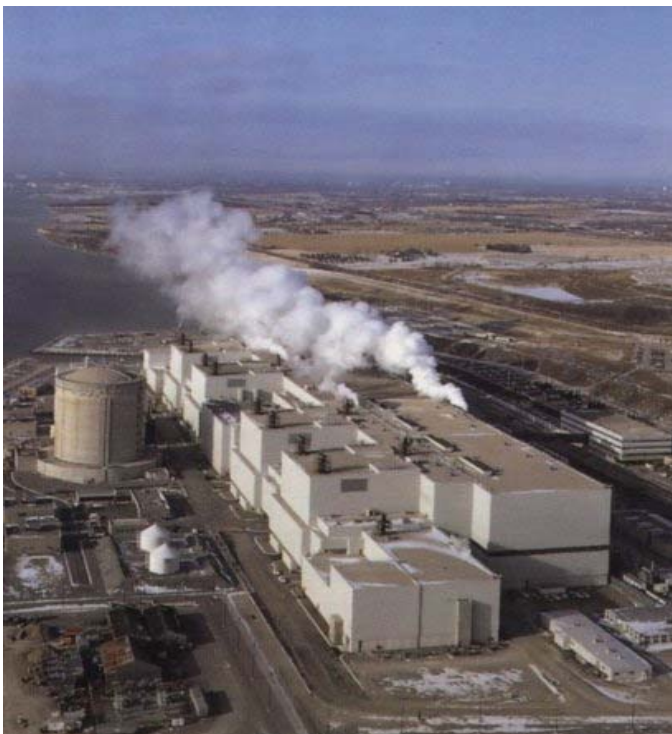
AECL's Darlington Nuclear Power Plant, Bowmanville, Ontario
